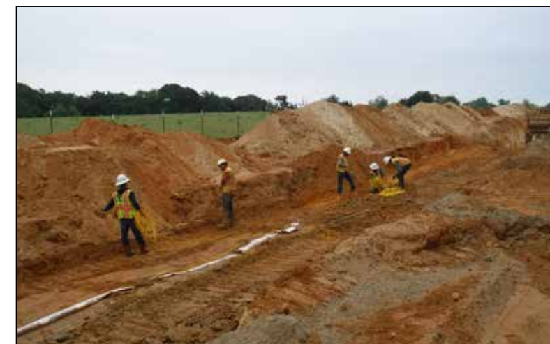
PL1011 Installing ribbon anode for cathodic protection to protect the IPL pipeline from the corrosive influence of other utilities
