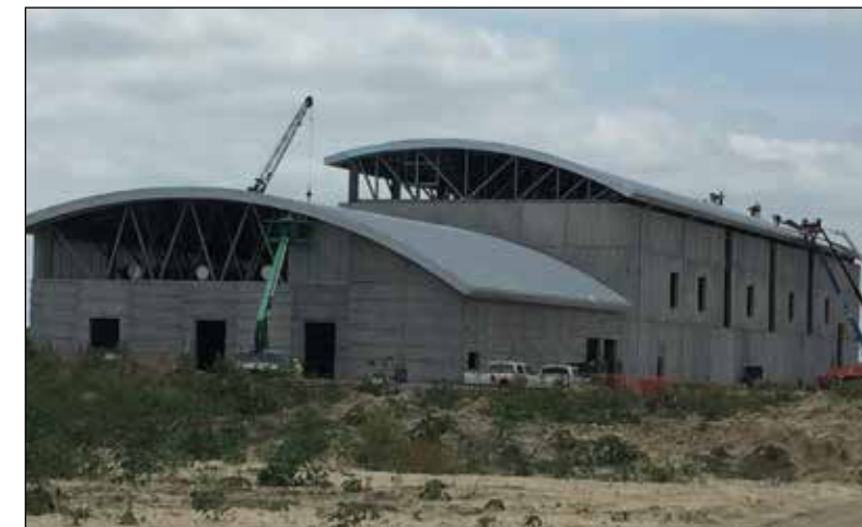
JB3 Pump Station roofing and exterior window panels installation
