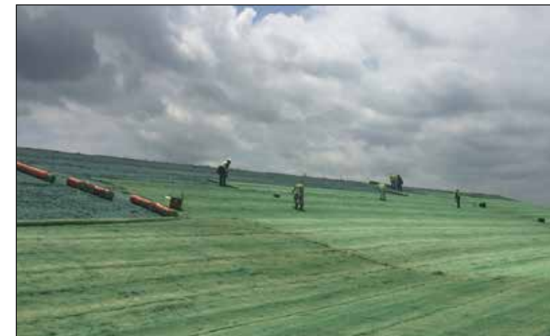
JB3RR Regraded and reseeded embankment slope of JB3 Reservoir
