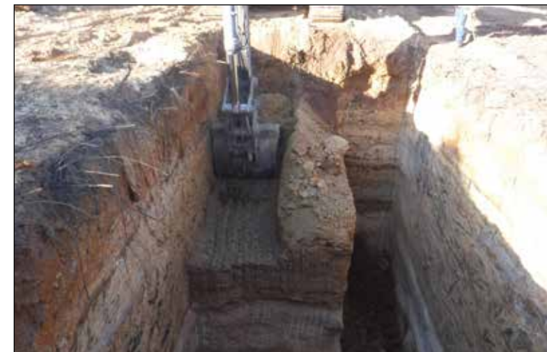
PL1011 Excavating launch pit for tunnel at Dick Price Rd.
