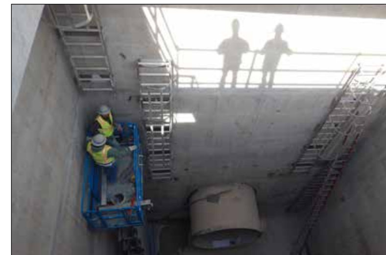
PL1213MBR Installing access ladders and platforms in 108-inch Gate Valve Vault
