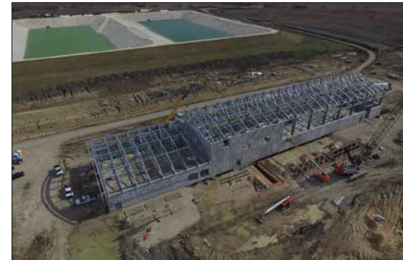
JB3 Aerial photo of progress at JB3 Pump Station
