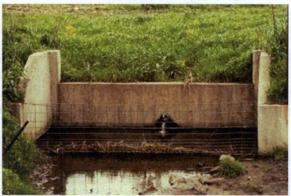
Figure 6. Grade stabilization structure (NRCS Online Photo Gallery)
